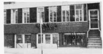
New York City Headquarters - RMC
