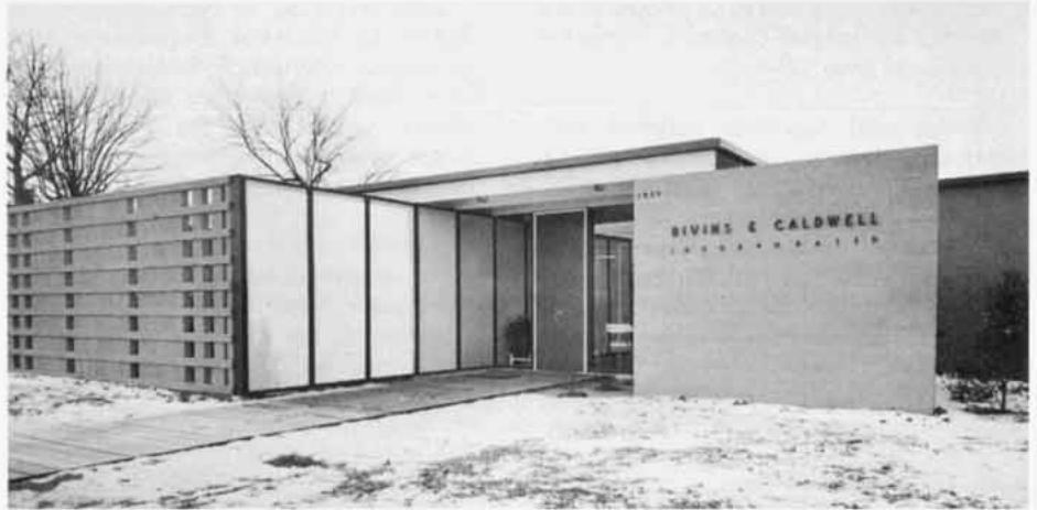
Headquarters of Bivins and Caldwell, Inc. in High Point, N. C.
