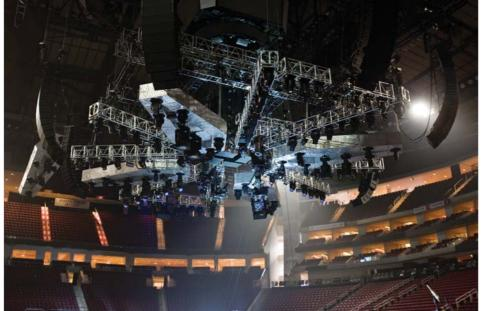
The innovative —and slightly odd-looking-P.A. features Meye Sound MILO and MICA loudspeakers, with 40 oo-HP subs around in four columns of 10. with all boxes turned so that the drivers are sitting together in the middle.
