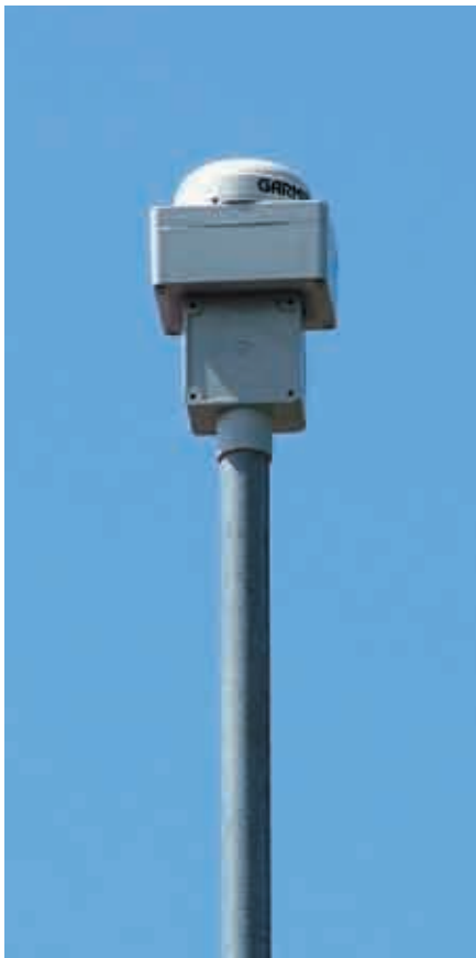
A small active GPS antenna is necessary to receive the GPS signals. The author used a Garmin GA 29 antenna. This was mounted on a plastic junction box and fitted to the top of an existing TV antenna mast.
