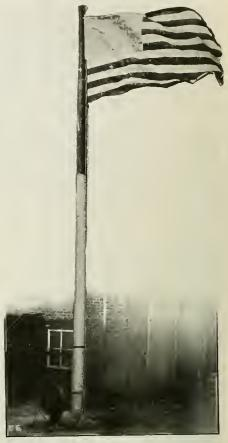
This Flag Always Waves, Whether There Is a Breeze or Not. A Motor-driven Blower Pumps a Strong Draft of Air Up Thru the Hollow Mast, Which Accounts for the Mysterious Effect Obtained.
