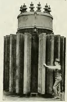
The Largest Self-control Induction, Voltage Regulator Ever Built.
