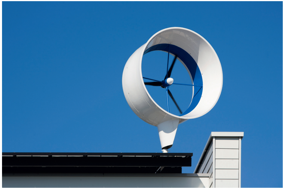
Figure 3.19 Small wind generator on a domestic property.
