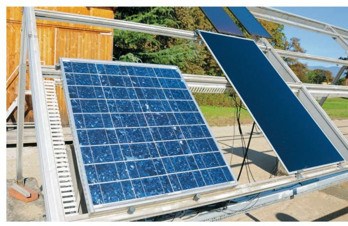
Roof not right for solar? No problem. Ground-mounting solves all sorts of logistical (and aesthetic) issues for both PV and solar thermal systems. Mounting racks can be purchased or built from scratch.
