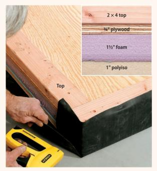
$13^{Construct the top from 2 \times 4s, \frac{3}{4}" plywood, \frac{1}{2} \text{ or } 2" \text{ rigid}}_{foam, \text{ and } 1" polyiso. Cut a 5' square of rubber liner for}_{the top, with 6" cutouts at each corner. Fold the flaps up the sides and over the top, then staple the rubber in place.}$
