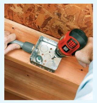
1 Mount a junction box inside the building where the conduit enters from the module. Secure the conduit to the box with appropriate connectors. Run two 14-gauge wires through the conduit, leaving excess at the module and junction box. OPTION: Using PVC conduit and electrical boxes instead of metal can reduce labor and materials costs and eliminate the need for grounding the metal conduit.
