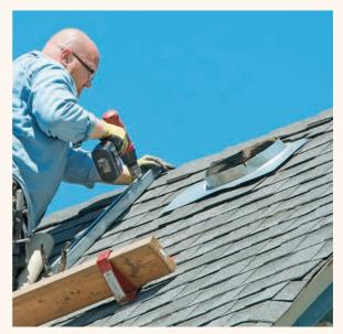
16 Attach Unistrut mounting U-channel bars to the roof for beach panel. Use the chalklines on the roof to determine the position of the Unistrut, and attach to the roof trusses with Unistrut connectors.
