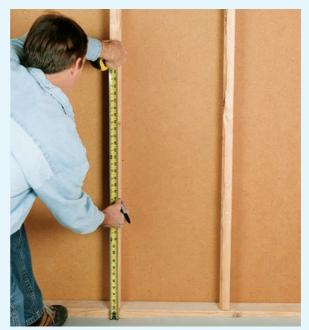
Plan the system layout. Determine the placement of the battery and then decide where you will position the charge controller and DC disconnect. The battery should be placed at least 18" off the ground in a well-ventilated area where it won't be agitated by everyday activity. Mark locations directly on the wall.
