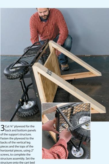
and mark the locations for four or more mounting bolts. Remove the structure and drill ¼" holes for bolts through the plywood base and bottom support legs. Mount the structure to the cart with 3½" carriage bolts and nuts, using large washers to span the holes in the cart mesh.
