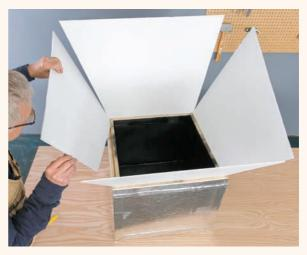
4 Lay out the reflector panels as shown in the Panel Layout drawing (page 105), using a yardstick, protractor, and marker. All of the four panels have the same width along the bottom, and both sides are angled outward at 67.5° toward the top. Cut out the panels with a utility knife. Test-fit all four panels by inserting their bottom edges all the way into the box channel grooves, and trim any panels as needed so they meet at the corners (it's not a problem if the corners have small gaps).
