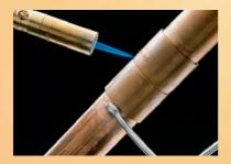
Heat the other side of the copper fitting to ensure that heat is distributed evenly. Touch solder to pipe. Solder will melt when the pipe is at the right temperature.
