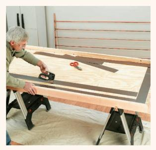
**9**Mark the manifold locations on the plywood, then cut 4"-wide pieces of aluminum flashing and staple them so they are centered under each length of copper. These will help transfer the heat to the copper pipes. Use stainless-steel staples.
