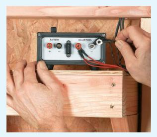
8 Connect the wires from the PV panels to the solar terminals on the back of the regulator/charge controller. Secure the wires to the walls or roof framing members to keep them clear. CAUTION: The collector panels should be covered with a drop cloth or opaque material well before making these connections. Tape or clamp the drop cloth so it doesn't blow off.
