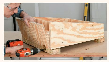
5 Glue and screw the hinged door pieces together, aligning the bottom and side edges, then set the door in position and screw on the hinges. Add a pull or knob at the center.
