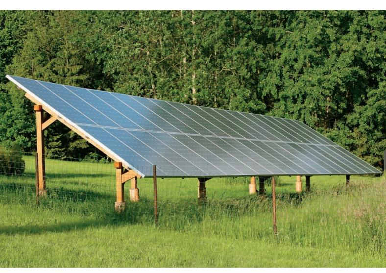
To protect against damage due to frost heave and ground movement, solar arrays must be set on poles that go down below the frost line. Some handy DIYers opt to use lumber for ground-mounting. Wood structures should be built with pressure-treated lumber and must be approved by the local building authority.
