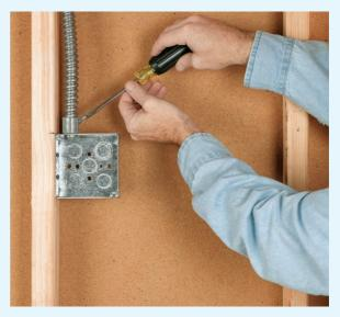
**4** Run flexible metal conduit from the entry point at the power source to the junction box for the DC disconnect box. Use hangers rated for flexible conduit.
