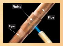
Move the torch flame back and forth and around the pipe and the fitting to heat the area evenly.
