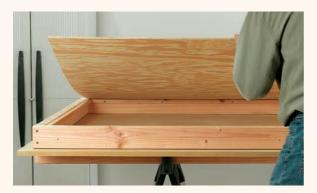
**3** Flip the frame over and set the ¼" plywood back into the frame against the nailers. Screw the plywood in place with ¾" machine screws driven through the back panel into the nailers.
