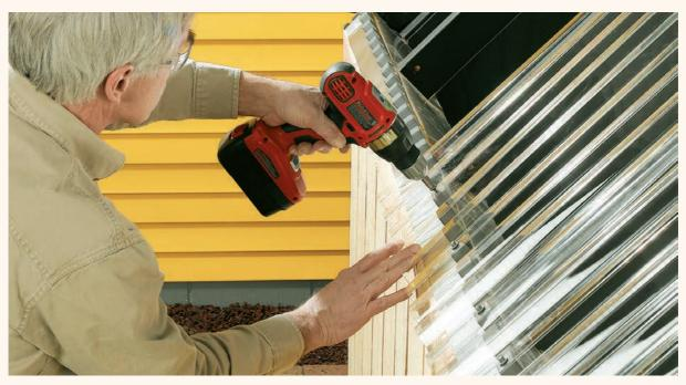
21 Set the panels in position over the foam closure strips, then predrill the holes on the crowns. Use a sharp bit <sup>1</sup>/<sub>6</sub>" bigger than the diameter of the neoprene screw to allow for movement. Don't overtighten the screws—they should be tight against the panel, but should not distort it.
