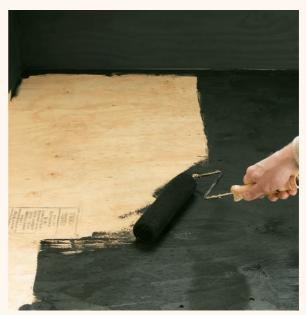
**19** Paint all of the interior with black roofing paint. Caulk all the corners with black silicone after the paint dries. Paint or stain the exterior whatever color you wish, but use acrylic latex so any trapped moisture can escape.
