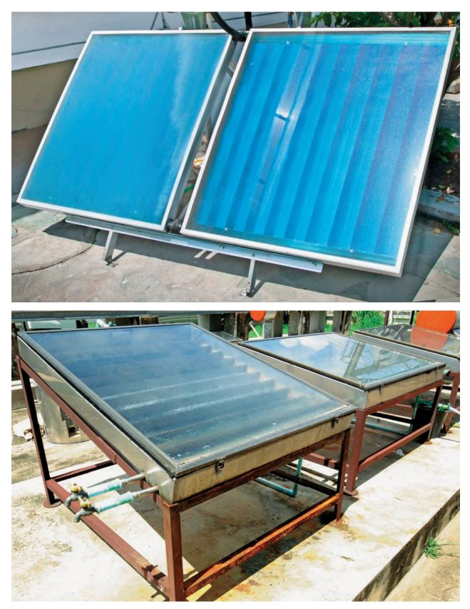
Solar water heating systems can heat water for domestic use (drinking, showering, etc.) or for water-based space heating systems. In both cases, the solar system typically preheats the water and a conventional water heater or boiler takes it from there. Commercial hot-water systems (top) save fuel, although the cost savings vary. DIY systems (bottom) can offer better payback potential.
