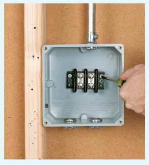
**8** Mount a PVC junction box for the battery controller about 2' above the battery location, and install two insulated terminal bars within the box.
