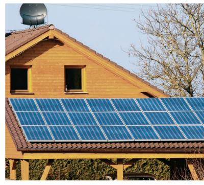
If your house already has power lines coming in from the utility company, it makes sense to leave them connected when you install solar panels so you can use the electrical grid for storage and backup.
