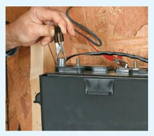
**9** With the regulator turned off, fasten the battery leads to the back of the regulator, then clamp them to the battery posts black to negative first, then red to positive. Then uncover the PV panels. Double-check the connections, then turn the regulator/ charge controller on. For a 12V battery, the voltage output reader will show 13 when the battery is fully charged.
