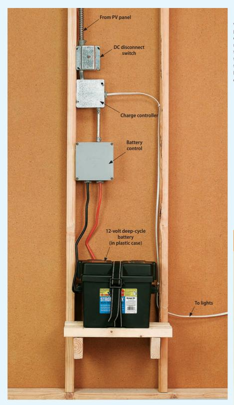
**16**Cover all junction boxes. Wires at the solar module to the positive and negative terminals on the module. When you're ready to test the system, remove the cover from the module, and turn on the DC disconnect switch to complete the circuit. Test the lights and adjust the time to the desired setting.
