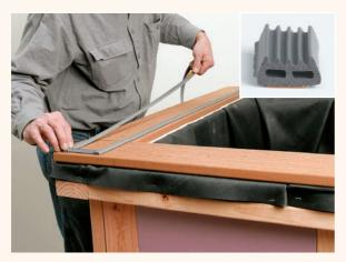
16<sup>Add</sup> two strips of weatherseal on the ledge about 2" apart. Use a soft foam type that compresses easily and fills voids, like this (inset).
