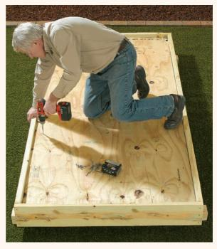
$2^{\mbox{Flip}}$  the framework over, then screw  $\frac{1}{2}$  " treated plywood to the underside of the frame. Caulk all the edges to prevent ants and other insects from colonizing the base.
