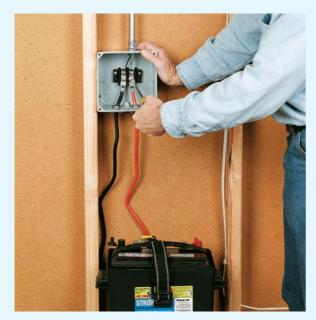
14 Install the battery. Here, a deep-cycle 12-volt marine battery is used. First, cut and strip each of the two battery cables at one end and install into the battery control junction box through cord cap connectors. Terminate these wires on two separate, firmly mounted insulated terminal blocks.
