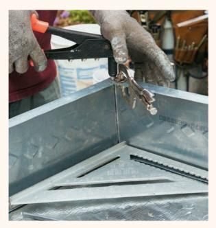
$\label{eq:steps} B^{\text{Fasten}} \ \text{the corners of the metal box with two $\%$"-dia.} \\ \text{Sheet-metal pop rivets in the top and bottom. Leave one corner open to create access for the insulation panel insert.} \\$
