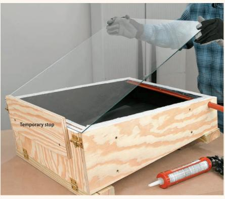
12<sup>Shim</sup> the box level and the top edge to make it easy to place the glass without smearing the caulk. Spread a generous bead of caulk on all the edges, then lay the glass in place. Tape it down around the edges with painter's tape, then let it set up overnight.
