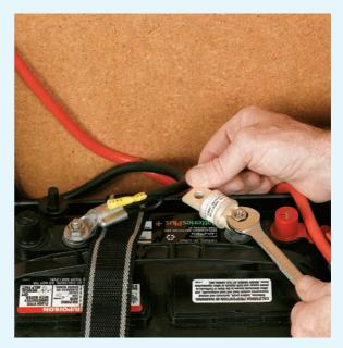
15 Install the catastrophe fuse onto the positive terminal using nuts and bolts provided with the battery cables. Connect the battery cables to the battery while paying close attention to the polarity (red to positive and black to negative). Make sure all connections have been made and double checked.
