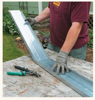
1 Cut and bend the box frame pieces from  $2 \times 6$  steel studs. Each steel stud piece will wrap two sides of the panel with a 90° corner bend. Mark the bend location on both steel studs. Cut a relief into the 6" side of the stud with aviation snips at this mark. Bend the stud to an L-shape and use a square to ensure that the corner forms a true 90° angle.
