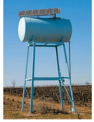
Water for irrigation is continuously pumped from a deep aquifer up to this storage tank during the day as long as the sun is shining.
