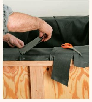
**1** Level out the rubber ledge between the corner folds with scrap pieces of rubber.
