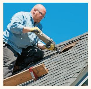
14 Mark off the panel layout locations on the roof. Transfer roof as well. The location of the 8"-dia. inlet and outlet holes to the roof as well. The location of these holes should not interfere with the structural framing members of your roof (either rafters or trusses). Adjust the panel layout slightly to accommodate the best locations of the inlet and outlet, according to your roof's setup. Cut out the inlet and outlet holes with a reciprocating saw.
