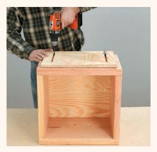
Screw the base and the plywood bottom together. Set the adjustable leg against one side of the base, then drill guide holes and install the hanger bolts so they will align with the slots. The centers of the bolts should be at the same height: roughly 2½" up from the bottom of the box. Use large fender washers and wingnuts to lock the adjustable leg in position.
