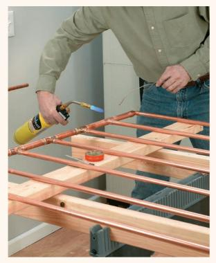
6 Solder all the pieces together. Protect the floor from drips of solder and flux with a dropcloth. Wait at least 5 minutes to touch the copper after soldering it—it will be very hot.
