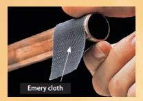
Clean the end of each pipe by sanding with emery cloth. Ends must be free of dirt and grease to ensure that the solder forms a good seal.
