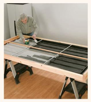
**1 4**<sup>Paint</sup> the entire inside of the collector with black, high-temperature paint.
