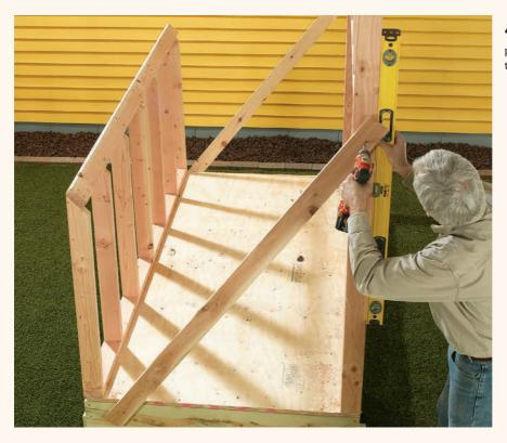
4 Frame the front and rear walls, then stand them up on the platform. Screw them in place, then level and brace the rear wall.
