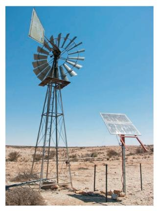
Once powered by a windmill that needed frequent maintenance, this deep well, which pumps water to a nearby stock tank, is now powered directly by solar modules. Instead of pumping on demand, the motor pumps water continuously when the sun is out and stores it in a large tank.
