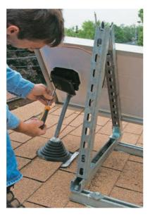
Connections for the feed wires that carry current from the collector are made inside an electrical box mounted on the back of the collector module.
