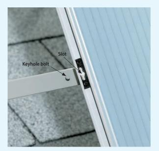
4 Lock the PV panel down into position by sliding the small bolt heads on the brackets into the keyhole slots on the back of the panel. (Other kits may use different fasteners.) Cover the panels with a drop cloth after they're in position-they'll start generating electricity as soon as the sun hits them.
