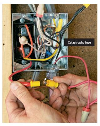
Remember to install all required fuses, charge controllers, and circuit breakers to ensure the safety of the system and the people using it.
