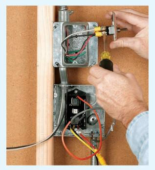
**1** Wire the DC disconnect. Attach the two #14-gauge wires to the two terminals labeled "line" on the top of the DC disconnect switch.
