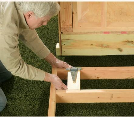
**1** Frame the rear doors. Make sure that the doors are ½" less than the height of the opening and ½" less (total) than the opening width. Frame openings for the vents, and add a hinge backer.
