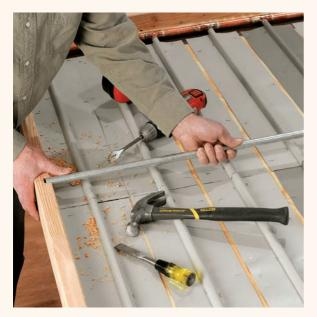
$12^{\text{Create cross-bar supports for the polycarbonate glazing} \\ \text{by installing two lengths of } \frac{1}{2}^{"} \text{ EMT conduit across the} \\ \text{box. Drill } \frac{3}{4}^{"} \text{ holes halfway through the } 2 \times 4 \text{ sides, centering the} \\ \text{drill bit } \frac{3}{4}^{"} \text{ down and drilling from the inside. Square the holes} \\ \text{with a chisel, then place the conduit in the holes.} \\ \end{array}$
