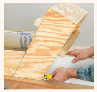
Line the sides and ends with 1" polyisocyanurate insulation. Leave the foil side facing into the box and glue the insulation in place with construction adhesive. Wrap the exposed upper edges with aluminum foil tape to protect the insulation from UV rays. Cut the insulation ¼" narrower than the plywood sides so that the bottom piece of ¼" plywood will fit in between the sides.
