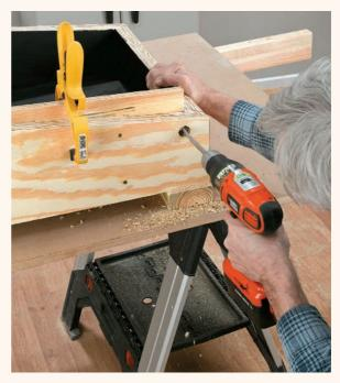
Brill a hole for the PEX drain. The top of the PEX is ½" down from the top edge. Clamp a piece of scrap wood to the inside so the drill bit doesn't splinter the wood when it goes through.
