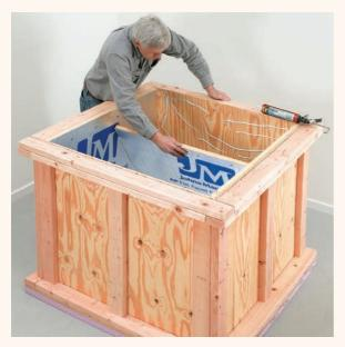
**Z**<sup>Place</sup> the polyiso insulation inside the box, using the foamboard adhesive to attach it. You don't need much; the water will hold the insulation in place. Add the second layer, then seal all the corners on the bottom and sides with silicone caulk.
