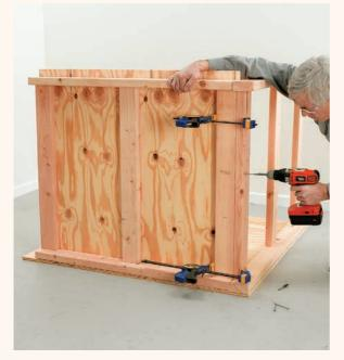
$\label{eq:stars} 3^{Place the \frac{3}{4}"} plywood base at the tank location, then connect the short sides to the long sides, fastening the overlapping corner 2 \times 4s together with the long deck screws.$
