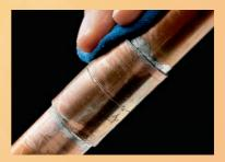
Allow the joint to cool briefly, then wipe away excess solder with a dry rag. *CAUTION: Pipes will be hot. If joints leak after water is turned on, disassemble and resolder.*
