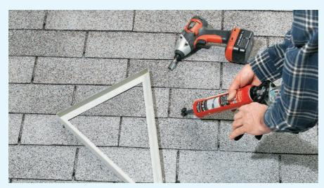
2 Predrill the holes for the mounting brackets (above), then fill them with roofing cement or silicone caulk (left). Fasten the brackets to the roof with neoprene screws (small lag screws with a rubber washer), or with toggle bolts if not attaching to a rafter.
