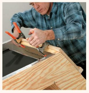
**O** Cut and install 1" polyiso insulation to fit the angled top, from the 2 × 2 to the outside corner. Caulk any gaps along the sides. Spread a bead of glue on the insulation, then cover it with 34" plywood screwed across the top, and extending from the 2 × 2 to 1" beyond the outside corner. Clamp the plywood and insulation until the glue sets.
