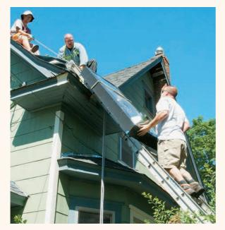
17 Hoist the panels into position. Carefully follow safety regulations and use scaffolding, ladders, ropes, and lots of helpers to hoist the panels onto the roof. Wear fall-arresting gear and take care not to allow the plenum ductwork to be damaged.
