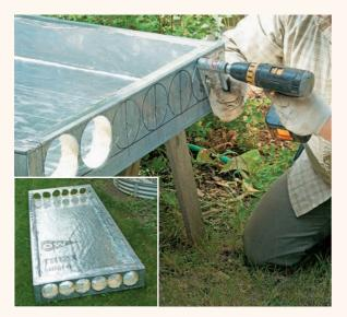
**Z**Create inlet and outlet holes in the walls with a hole saw or circle cutter. The number and location of the ductwork holes depends on where each panel fits into the overall array (presuming you are making and installing multiple panels). The first and last panels in the series will each have one end wall that is uncut, while intermediate panels will have duct holes on each end wall (inset).
