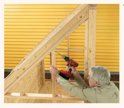
**1 O**<sup>Fill</sup> in the framing for the angled part of the sides.
