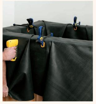
$10^{\text{Staple the rubber around the outside edge of the top}}_{2\times4\,\text{ledge.}}$
