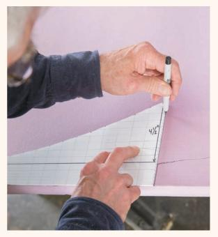
**6** Trace around the template to draw 16 ribs onto 1½" rigid insulation board, using a fine marker. Cut out the ribs with a jigsaw.
