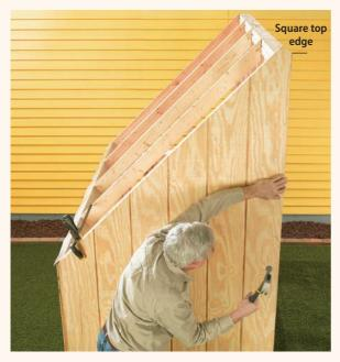
$12 \\ \text{Install exterior siding on the walls and doors and above} \\ \text{piece as shown so it lines up with the 2 \times 4 top plate and creates} \\ \text{a small roof profile.}$
