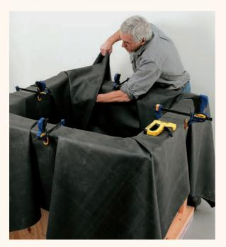
**9** Fold the corners as neatly as possible and clamp them in place. Don't stretch the rubber—leave it sagging at the bottom.
