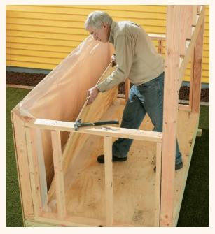
$Z^{\rm Insulate the front wall, then add the vapor barrier and the <math display="inline">\%"$  interior plywood siding. Leave the plywood % to %" short of the top plate.
