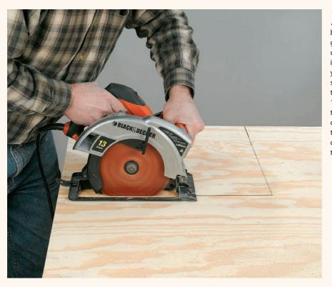
2 Lay a 4 × 8' sheet of plywood on the worksurface with the better side facing up. Select a good grade of <sup>3</sup>4" plywood (we used BC) or you're likely to have issues with parts warping, and you'll find it difficult to drive screws into the edge grain of the plywood. Mark and cut the  $19 \times 19$ " bottom piece first. Rest the full sheet of plywood on a couple of old 2 × 4s—you can cut through them as you make your cuts without any need to move them out of the way.
