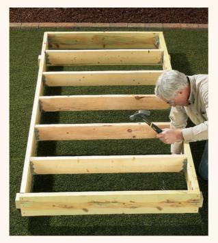
Level a base of treated wood or concrete blocks at the kiln location, then build the frame for the floor on top of them. The kiln should be built in a south-facing location that gets at least five to six hours of direct sunlight.
