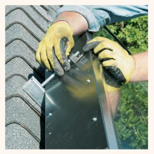
**19**Connect the panels to the Unistrut with a <sup>3</sup>/<sub>6</sub>" threaded outside. Cut threaded at the top and bottom of the panel on the Unistrut nuts. Attach the top clip to the top of the rod and the front face of the panel. Tighten the assembly to compress the panel down to the Unistrut for a tight hold.
