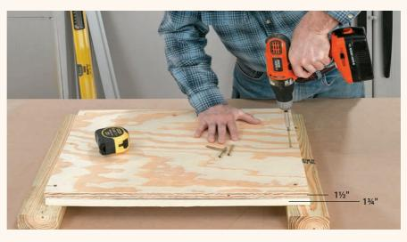
3 Screw the first layer of front and side pieces to the base and to each other, then add the back piece. Predrill the screws with a countersink bit.
