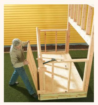
6 Nail the exterior siding to the framing for the front wall. The top edge should be lower than the top of the 2 × 4 framing to leave room for the glazing overhang. Nail temporary stops at the corner to help position the siding.
