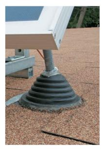
An EPDM rubber boot seals off the opening where the PVC conduit carrying the feed wires penetrates the roof.
