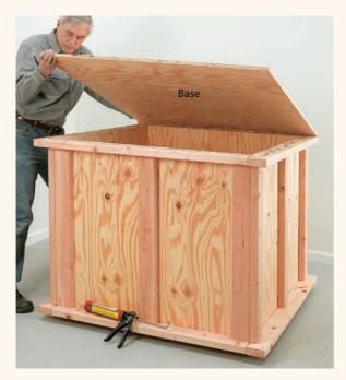
5 Tip the box over, then glue and screw the plywood base to 5 the 2  $\times$  4 frame, aligning all the edges.
