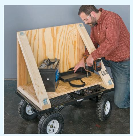
4 Install the module mounting brackets onto the support legs, using 1½" screws, then test-fit the module. NOTE: Leave the module covered with a tarp for safety; it will produce power even when exposed to artificial light. Determine the positions of the system components, including the battery, and mark the locations of holes for wiring runs through the plywood back panel. Also drill a hole through the base panel for a bonding wire between the bus bar and the cart bed.
