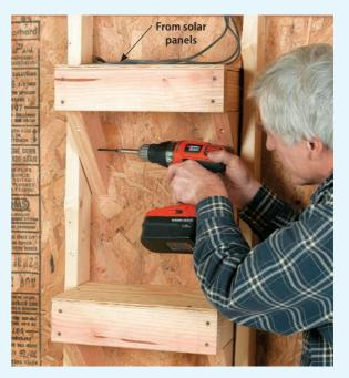
Z Install two sturdy shelves inside the building to hold the regulator and the battery. The shelf should be reachable by an adult so the equipment can be turned on and off and plugged into the adapter easily. The battery shelf should be at least 18" off the ground.
