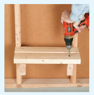
${f 9}^{Build}$  a support shelf for the battery using 2 × 4s. The shelf should be at least 18" above ground. Set the battery on the shelf in a sturdy plastic case.
