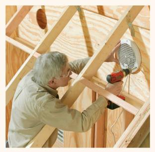
1 **Z**Fasten the fans to the shroud. The fans are turned on during the day to circulate the air, then turned off at night so the wood doesn't dry too quickly, so they should be plugged into a timer.
