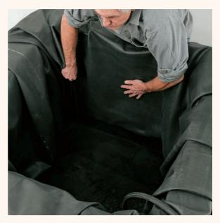
Out and set aside a  $5 \times 12'$  piece of the EPDM for the top, then fold the remainder into the tank. Work it into the corners, leaving the rubber loose at the bottom so it doesn't stretch with the weight of the water. Add 6" of water to hold the rubber in place as you fold over the corners. Drape the excess over the sides.
