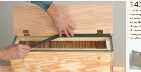
14 Cut 1 × 8s to fit for covers for the inlet and outlet, so that heat won't be lost when the sun goes down. Apply selfadhesive weatherseal around the edges, then screw on two or three hinges, depending on the width of the window. Use hooks to hold the upper cover in place and small barrel bolts to hold the lower cover.
