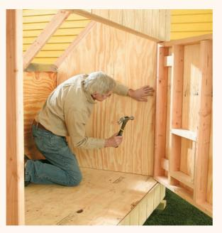
Add insulation to the walls and doors, staple on the vapor barrier, then nail on the interior plywood siding.
