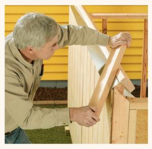
Nail the coil stock to the top plate, leaving a 3" overhang on each side. Screw a 2 × 4 over the coil stock, matching the top plate position, then bend the coil stock over the edges and nail it in place. (Gutter repair tape or a strip of EPDM roofing can be used instead of coil stock.)
