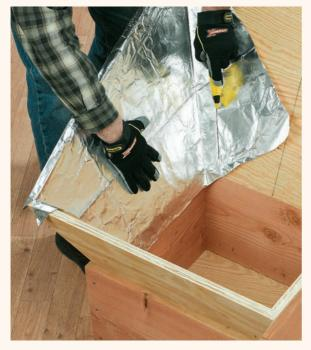
**10**<sup>Cut</sup> pieces of reflective sheeting to fit the sides of the reflector as well as the base. You can use heavy-duty aluminum foil, but for a sturdier option try solar foil (see Resources, page 186). The product seen here is essentially polyethylene tarp material with a reflective aluminum surface. Make sure to cut the pieces large enough so they overlap the edges and can be easily attached.
