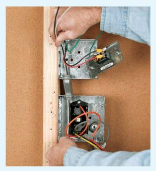
Z Install the charge controller inside the double-gang box. Run flexible conduit with connectors and conductors from the disconnect box and to the charge controller box.
