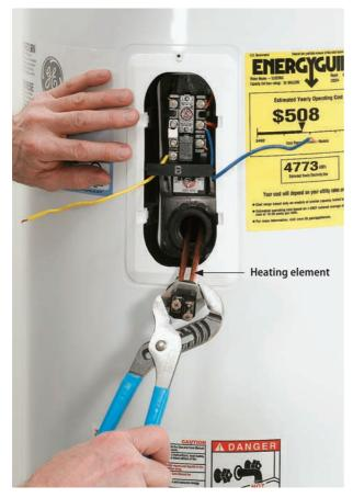
Turn off and disconnect any wiring to the heater you'll be converting to a storage tank. Remove the covers over the heating elements, cut away the wiring, then turn out both heating elements with a socket wrench or a channel lock wrench.
