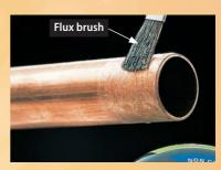
Apply a thin layer of soldering paste (flux) to the end of each pipe, using a flux brush. Soldering paste should cover about 1" of pipe end.
