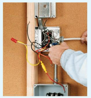
12 Run wiring to the loads (exterior DC lighting fixtures in this case) from the charge controller. DC light fixtures (12-volt) with LED bulbs can be purchased at marine and RV stores if you can't find them in your home center or electrical supply store.
