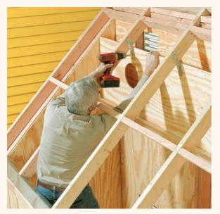
**16**<sup>5</sup><sup>2</sup><sup>4</sup> Plywood. Attach 2 × 4 nailers to the sides (hidden behind the shroud in this photo), and screw a 2 × 4 across the bottom. Make cutouts for the fans you buy, then hang the shroud from the rafters with hurricane ties and screw the 2 × 4 to the side walls. (Fans can be any inexpensive type, 8" to 14" round or square, as long as you can find a way to fasten them.)
