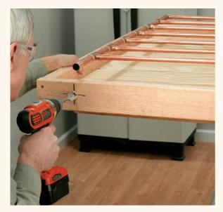
8 Mark the location of the cold-water inlet and the warm-water outlet on the sides of the box by setting the copper grid into the box and extending the inlet and outlet port locations onto the outside of the frame. Drill the holes with a 1"-diameter bit.
