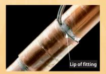
When solder melts, remove the torch and quickly push  $\frac{1}{2}$ " to  $\frac{3}{4}$ " of solder into each joint. Capillary action fills the joint with liquid solder. A correctly soldered joint should show a thin bead of solder around the lips of the fitting.
