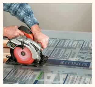
**1** Ocut the polycarbonate glazing so that it matches the width of the box. Cut it long enough so it tucks under the overhang at the top and hangs over ½" at the bottom. Make sure to install it with the UV-protected side up (the side with the label).
