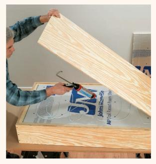
Turn the box over, add the 1" insulation to the bottom of the box, then cover it with the  $\frac{1}{2}$  plywood. Glue the plywood to the insulation and screw it to the 1 × 3 nailer with 2<sup>1</sup>/<sub>4</sub>" screws.
