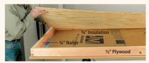
4 Cut panels of ¾"-thick closed-cell, foil-faced polyiso insulation and fit them inside the frame between the ¾" nailers, flush with the tops of the nailers. Cut a panel of ½" plywood to fit inside the frame over the insulation and the nailers and attach the plywood to the nailers, driving a 1¼" screw every 10" to 12" around the perimeter. Caulk the gap between the ½" plywood and the frame with clear, 100% silicone caulk.
