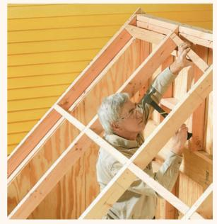
$15^{\text{Attach crosspieces between the rafters to stiffen and}$  support the glazing panels. Screw them in through the backs of the rafters at an angle.
