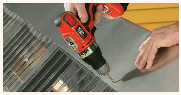
22<sup>Cut a 14"-wide piece of sheet-metal or aluminum coil stock slightly longer than the roof, then bend it at the center to create a cap for the roof. Drill holes through the metal, polycarbonate, and closure strips in the front, then fasten with neoprene screws into the blocking. Screw the metal to the 1 × 6 in back.</sup>
