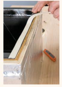
Plave a piece of ¼" glass cut to 17¼" square. Ask the glass supplier to sand the sharp edges, or sand them with 100-grit sandpaper. Attach metal door pulls designed for glass doors as handles for the sides of the glass. (You may need to buy these at a woodworking or cabinet supply company.) When using the cooker, use these handles to insert and remove the glass in the cooker.
