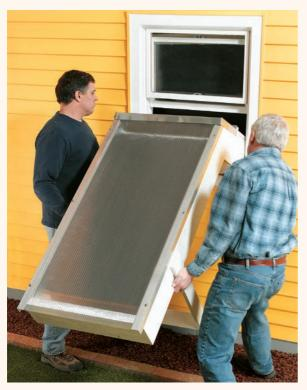
1 5 Set the solar collector in the window with the pushed against the sill (you'll need a helper for this). Fasten  $1 \times 3$  supports to the sides, then screw them to the house with metal angle brackets or a  $2 \times 4$  between the supports. Attach the collector to the window sash on the inside with small angle brackets placed on the  $2 \times 2$ . Wedge foam backer rod or other type of weatherseal into gaps around the window jamb and into the gap between the upper and lower sash.
