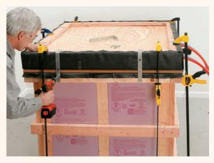
17 Complete the plumbing connections inside the tank, fill gaps around the pipes on the ledge with silicone, then clamp the top down tightly to seal the edges. Fasten the top to the base with galvanized straps and deck screws.
