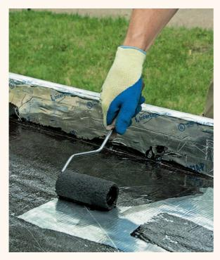
**9** Paint the entire box interior using black high-temperature paint and allow it to dry completely. A trim roller works well for this task.
