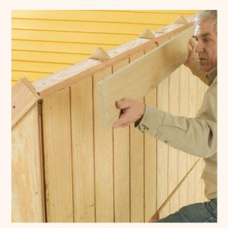
$18^{Form the top of the kiln by extending the 1 \times 4 diagonal trim to the edge of the framing, then join the two sides of the kiln with a 1 \times 6 cap. Nail on triangular blocks for nailers and to help support the peak of the roof.}$
