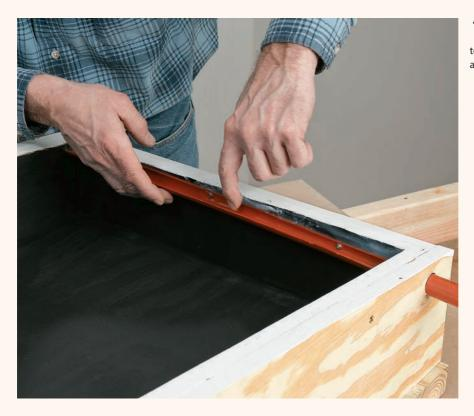
**1** Wipe a thick bead of silicone caulk along the top edge of the PEX to seal it against the plywood.
