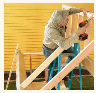
**9** Measure and cut the rafters. Lay out the rafters 24" on center, starting with the center rafter and working to the sides, so that the overhang at the edges will be equal. Check the rafter layout against the polycarbonate panels to make sure they line up properly. Note that the panels are fastened through the crowns, rather than in the valleys.
