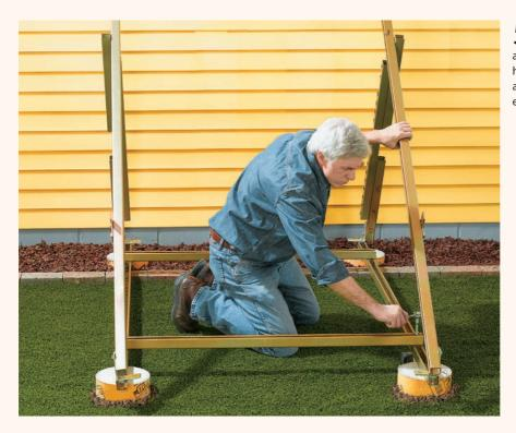
**5** Although the PV mount is stable, it needs to be securely anchored to the ground in case of high winds. For larger arrays such as ours, add concrete footings at each corner.
