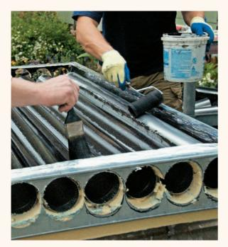
Paint the last section of ductwork and touch up around the interior of the box so all exposed surfaces are black.
