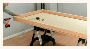
1 The frame that houses this solar water heater is constructed from  $2" \times 4"$  and  $2" \times 6"$  dimensional lumber. Cut the pieces of the frame to length, then join them with  $2\frac{1}{2}"$  deck screws driven into pilot holes.
