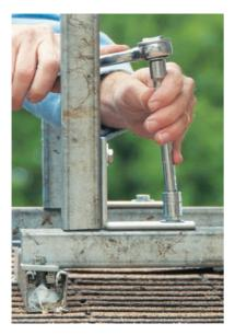
The stand components are held together with bolts and spring-loaded fasteners. The 45° and 90° connectors are manufactured specifically for use with this Unistrut system.
