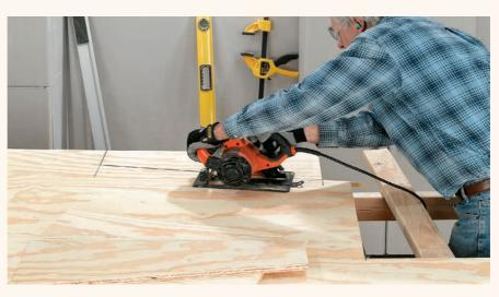
$2^{\text{Cut the insulation the same}}_{\text{size as the plywood base, then}}_{\text{screw both to the 2 \times 4 supports}}$  with 2½" screws.
