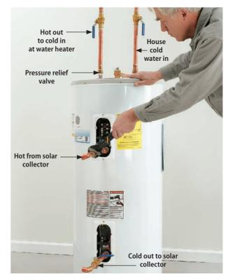
Solder several inches of  $\frac{3}{4}$ " pipe to 1"  $\times \frac{3}{4}$ " reducers so you don't have to use the torch near the plastic and insulation in the water heater. After the pipes cool, wrap the fittings with teflon tape, then thread them into the water heater. Tighten with a wrench, then connect to the PEX lines coming from the solar collector. Connect the house cold water supply to the cold inlet at the top, then connect the hot output to the cold inlet at the main hot water heater.
