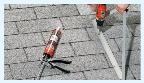
1 Locate the roof rafters, either by using a stud finder or by lifting up shingle tabs and tapping in finish nails. You must plan to fasten at least one of the angled mounting brackets to a rafter. If the other doesn't fall on a rafter, plan to attach it with toggle bolt anchors.
