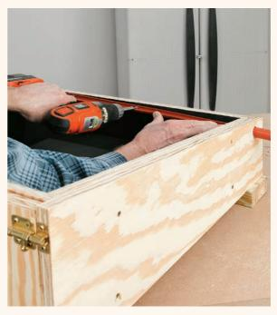
$10^{\text{Drill three } \%"} \text{ holes in the side of the PEX for screws, then} \\ \text{other side, the PEX through the hole. Butt it tight against the other side, then screw it in place, sloping it about <math>\frac{1}{4}$ ".
