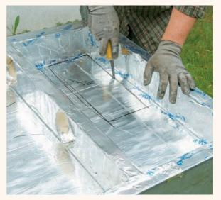
Binstall a compartment separator in the first and last panels with a piece of foil insulation set on edge. Cut ductwork access holes in the separator. Then, cut out holes for the ductwork that will pass through the separator. Also cut a plenum opening in the separated compartment in the first and last unit.
