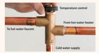
Install the tempering valve on the hot water line after it comes out of the heater, before it goes to any fixtures. Connect it to the cold water line. Then reconnect the hot water supply for the house fixtures to the outlet marked "Mix." If you buy a valve with sweat connections, remove the knob and the thermostatic controls inside the valve before soldering, then reinstall them when the pipes are cool.
