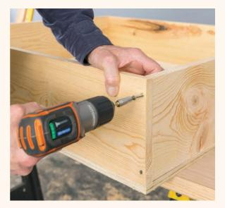
$4^{\text{Cut}}$  two pieces of 1" × 8' to length at 36" and two pieces at 37½". Apply construction adhesive to the bottom edges, and glue the boards along the edges of the top face of the plywood base, so the longer pieces cover the ends of the shorter pieces. Drill pilot holes, and screw the boards together at the corners, using 1½" screws. Also fasten the boards with screws driven through the bottom of the base.
