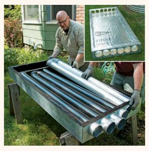
**1** O<sup>Insert</sup> the ductwork. Beginning at the inlet duct, guide 4" aluminum HVAC ductwork in a serpentine shape throughout the entire multi-panel installation, ending at the outlet duct. Join ends of adjoining duct sections with flexible duct connectors fashioned into a U shape and secured with metal screws and foil tape. Paint each section of ductwork with black high-temperature paint once it is in place.
