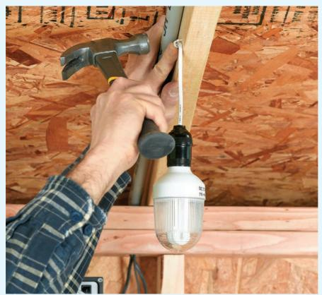
**10** This kit includes two DC lights. To install them (or other DC appliances), just plug the cord in to the proper port (or adapter) and turn the power on. Hang the 12-volt light fixtures from the rafters and then staple the cords to keep them secure and out of the way. Make sure to leave enough cord that the plug end is easy to insert and remove from the port. You'll plug and unplug the lights to turn them on and off.
