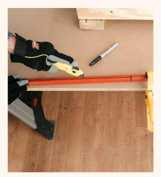
**9** Mark the first 19" of PEX, then cut it in half with a utility knife. Score it lightly at first to establish the cut lines.
