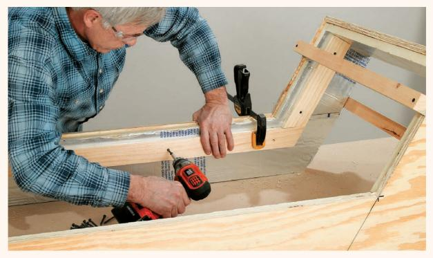
**5** Screw the  $1 \times 3$  nailers to the sides of both the long and short pieces using  $2\frac{1}{4}$ " screws. Place the nailers  $1\frac{1}{4}$ " from the bottom edge to leave room for 1" insulation and  $\frac{1}{4}$ " plywood.
