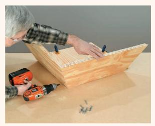
6 Assemble the reflector. Brace two of the reflector sides against a square piece of scrap plywood clamped to the work surface, then join the edges with screws driven into countersunk pilot holes. Repeat for the other two pieces, then join the two halves together with four screws at each corner, completing the reflector. The bottom edges should be aligned. The top edges won't match perfectly, so sand them smooth.
