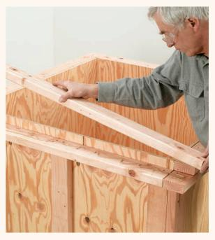
**6** Glue the 2" foam base to the plywood base with construction adhesive, then turn the box right-side up and add the second layer of  $2 \times 4s$  to the top, overlapping the corners for strength. Screw the plywood walls to the final layer of  $2 \times 4s$ .
