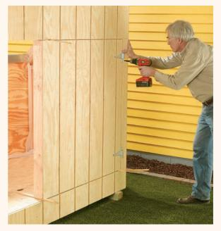
$13^{\rm Screw the strap hinges to the doors at the 2 \times 4 backer locations. Shim the doors so they're tight and evenly spaced in the opening, with the door against the frame, then screw the hinges to the frame. Drive just one screw into each hinge at first, then remove the shims and check the fit. Adjust if necessary when you drive the rest of the screws in.$
