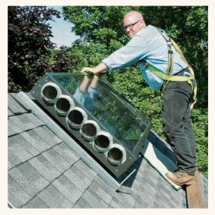
20 Seal the panel connections with 1" foam gasket tape around each end of the panels where they connect. Place a bead of silicone caulk on top of the gasket tape and then attach 3"-wide flashing over the two panels at the joint. Attach flashing to the panel with galvanized sheet-metal screws with rubber gasket heads.
