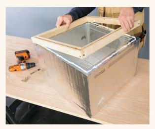
**3** Complete the box by cutting four pieces of 2 × 2 channel to length at 19", mitering the ends at 45°. Glue the pieces to the top edges of the box sides with foamboard adhesive so all of the beveled grooves angle outward from the box center and they meet at the corners. Let the adhesive cure, then paint the interior of the box with black spray paint.
