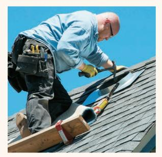
15 Use a roof jack to form an 8"-dia. opening. Apply a heavy double bead of roofing cement along the top and sides of the jack. Nail the perimeter of the flange using rubber gasket nails. Cut and install shingles with roofing cement to fit over the flashing so they lie flat against the flange.
