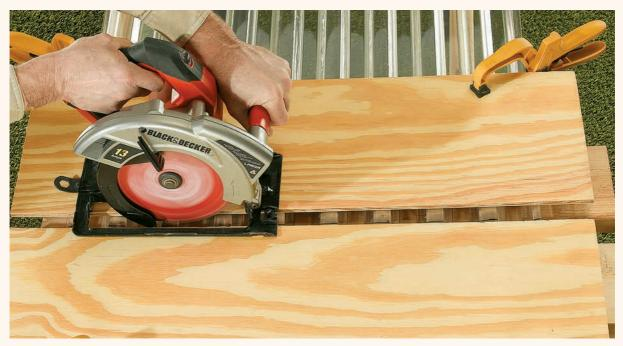
20 Align the four polycarbonate panels, then clamp the ends with spring clamps and mark the cut line. Place 2 × 4s under both spring clamps of the cut, then place cardboard or plywood on top, under the circular saw, so the panel doesn't get scratched. Use a sharp plywood-cutting blade (or whatever blade the panel instructions recommend) to cut the panels.
