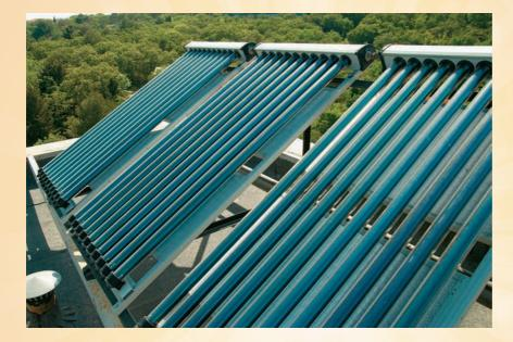
Evacuated-tube collector: This type of collector has to be purchased from a supplier, although homeowners can install it. Water pipes in this system, instead of running through an insulated box, are installed inside a round tube of insulated glass. The vacuum inside the insulated glass allows light through, but slows heat loss. Evacuated-tube collectors are more efficient than flat-plate collectors in partially sunny or cloudy conditions.
