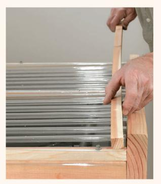
$16^{\text{Cover the ends of the glazing with }\frac{3}{2} \text{ wood strips. Predrill}} \\ \text{and fasten the strips with }\frac{2}{2} \text{ deck screws. Caulk the strip} \\ \text{at the top against the } 2 \times 6 \text{ cap using paintable acrylic caulk.} \\ \text{Acressing paintable acrylic caulk } \\ \text{Acressing paintable } \\ \text{Acressing paintable } \\ \text{Acre$
