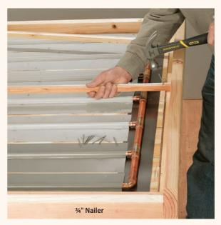
$13^{\rm A}$  Tay the glazing on top of the box and mark the spots for  $3^{\rm A}$  " nailers at the sides and the center overlap. Fasten the strips with 6d galvanized casing nails.
