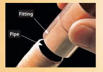
Assemble each joint by inserting the pipe into the fitting so it is tight against the bottom of the fitting sockets. Twist each fitting slightly to spread soldering paste.
