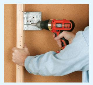
**3** Attach a junction box for enclosing the DC disconnect, which is a heavy-duty switch, to a wall stud near the battery and charge controller location. Use a metal single-gang box with mounting flanges.
