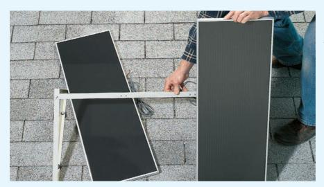
**3** Fit the bottom of the first collector module neatly into the slot in the mounting frame assembly.
