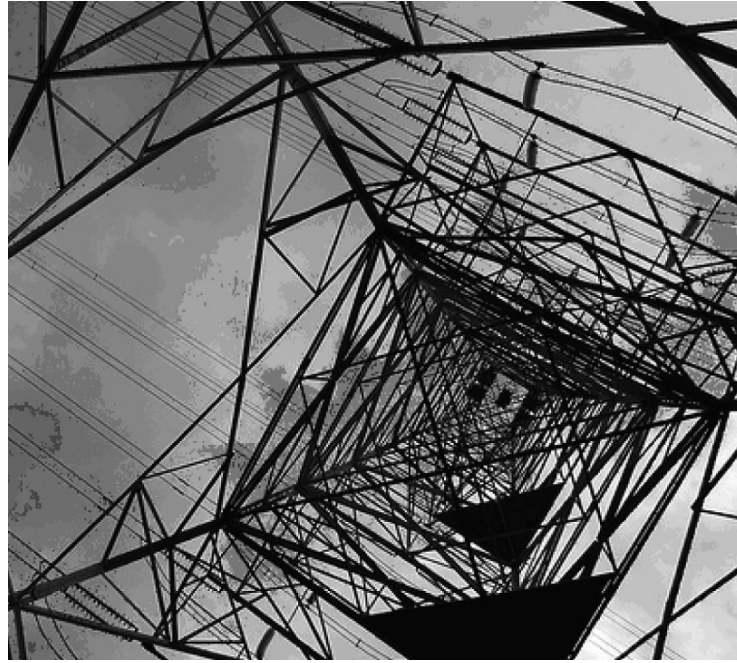
FIGURE 47.7 Steel lattice structure of a transmission line tower.
