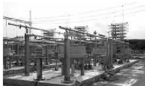
FIGURE 31.28 Installation of the triple-tuned filter at the Gurun station in Malaysia.
