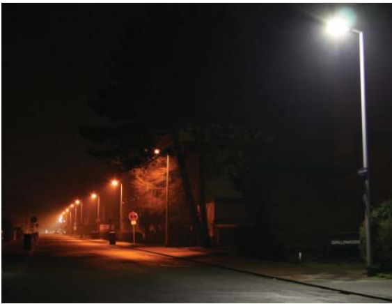
Figure 8.15 An S4-class street in Darmstadt, Germany, illuminated partly by white high pressure mercury luminaires at 4000 K and partly by yellowish-orange high pressure sodium luminaires. (Photo Source: Technische Universität Darmstadt.)
