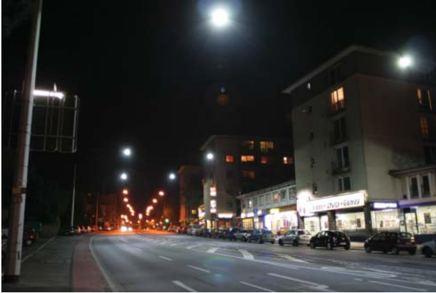
Figure 8.14 An ME2-class main street in Darmstadt, Germany, illuminated partly by cool white LEDs at 5700 K and partly by yellowish-orange high pressure sodium luminaires. (Photo Source: Technische Universität Darmstadt.)
