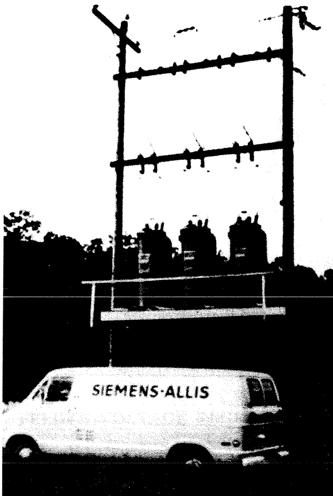
FIGURE 9.4 Typical platform-mounted voltage regulators. (Siemens-Allis Company.)
