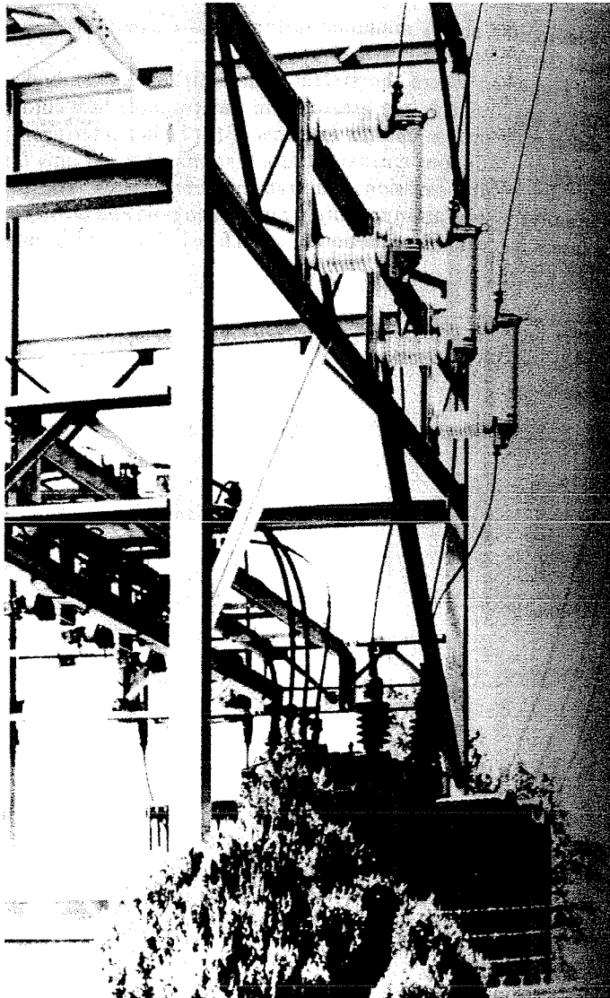
FIGURE 10.6 Typical transformer protection application of 34.5-kV solid material-type power fuses. ( S&C Electric Company .)
