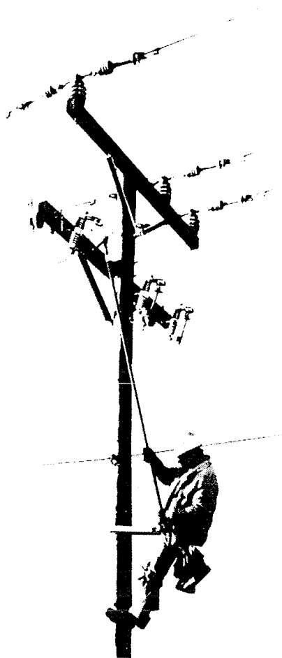
FIGURE 10.3 Typical application of open-fuse cutouts in 7.2/14.4-kV overhead distribution. ( S&C Electric Company. )
