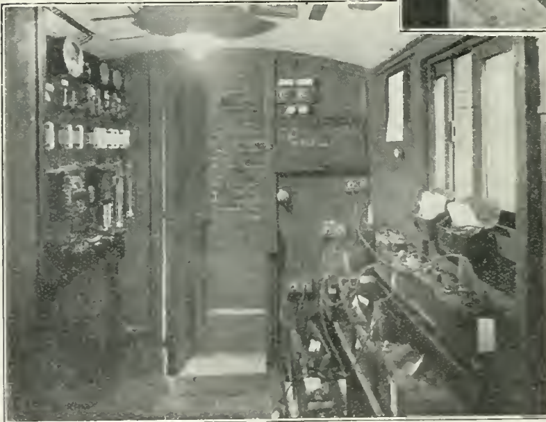
Above. — The motor generator and main switch-board at the charging station of The Park Motor Co., Ltd., in Wells Street, S.W.
