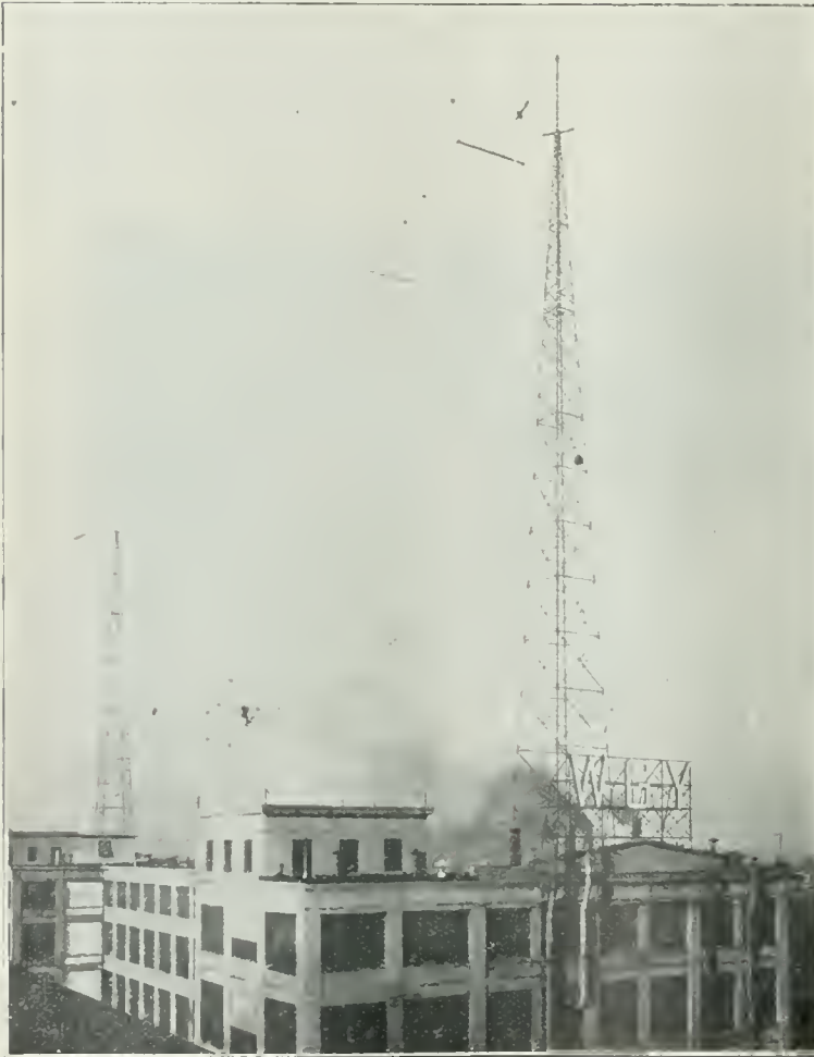
A general view of the antenna system of the American Broadcasting Station, WGY, at Schenectady, N. Y.
