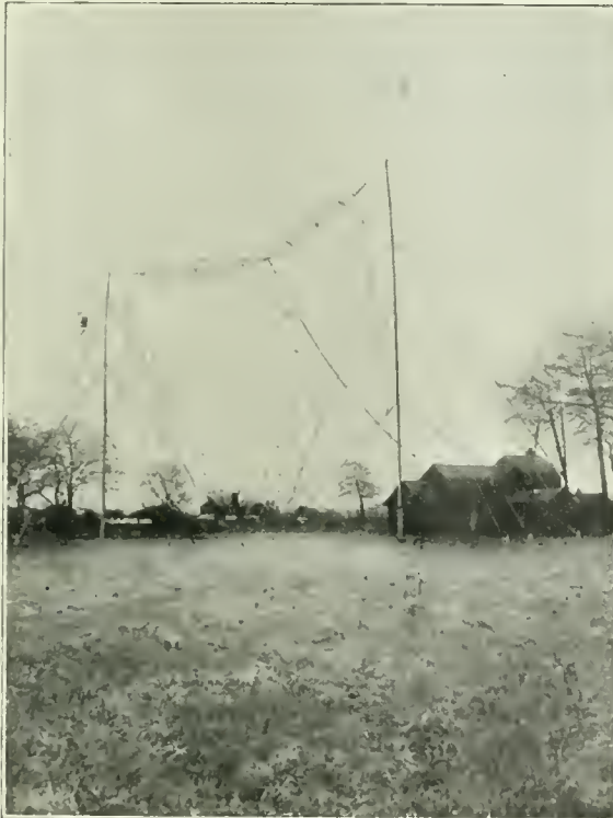
The aerial. It is 80 ft. high and the masts are 120 ft. apart.
