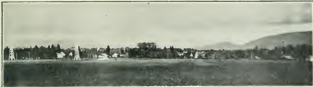
General View. The Aerial and Transmitting Building are on the left and the Hangars on the right.
