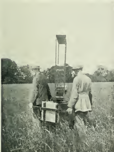
Fig. 4a. Photograph showing mode of carrying the D.F. set without dismantling.
