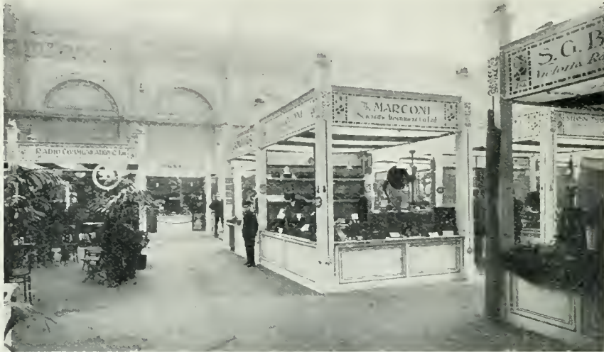
A General View showing some of the Stands.
