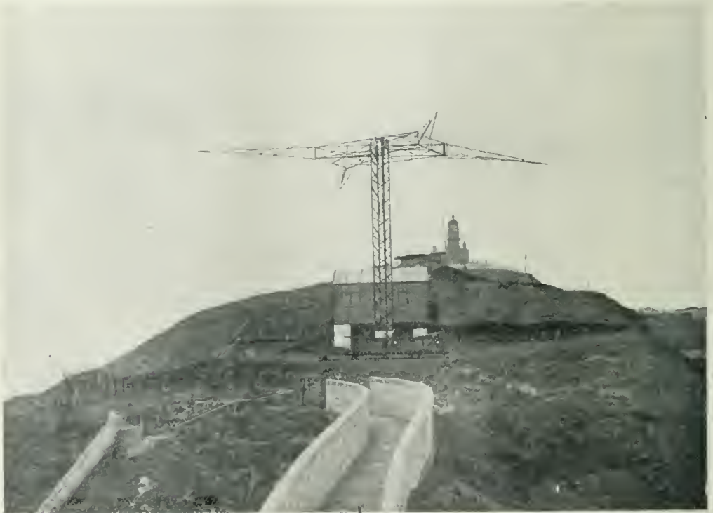
Fig. 106. The Parabolic Reflector at Inchkeith, Firth of Forth, Scotland, as used for directional short wave wireless telephony.
