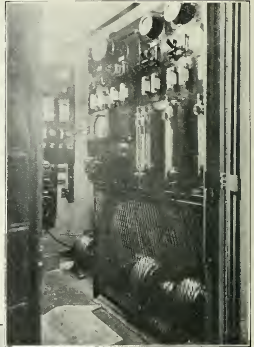
Above. — The motor generator and main switch-board at the charging station of The Park Motor Co., Ltd., in Wells Street, S.W.
