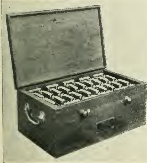
Chloride 30-Cell 60-volt AYGI type batteries.
