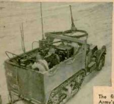
ing specifications necessitated by its work as a mobile radio. It is a 450-watt voice and C.W. set, which had been thoroughly tested and proved as an amateur rig before be-ing drafted into the service of the country. It is powered —as are the receivers and an electric heater also in-stalled in the truck—by a 117-volt Onan generator in a trailer behind the truck. The equipment includes two stanequipment includes two stan-(Continued on page 701)
