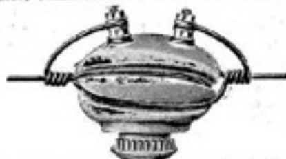
This Novel Insulator Has Fuse Plug Inside.
