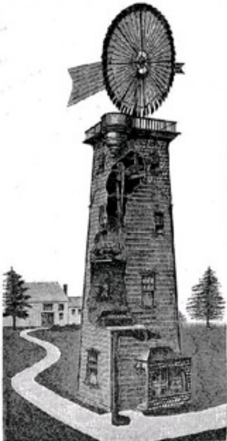
Windmill Drives Electric Lighting Dynamo and Charges Also a Storage Battery.
