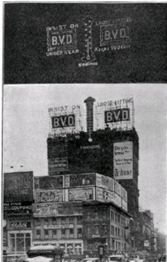
Novel New York City Electric Sign Which Tells the Public the Exact Temperature at Any Time, Day or Night, by Means of Electric Lamps.
