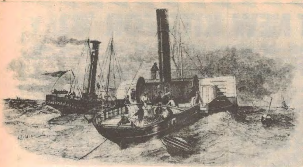
First underwater telegraph cable between England and France, shown here being laid by the tug Goliath, August 28, 1850.
