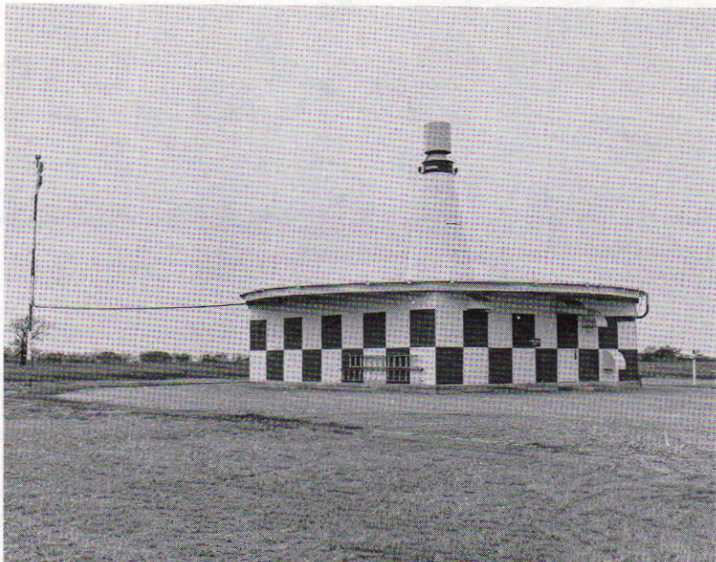
Fig. 1-12. A typical VOR station.
