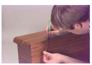
12. Once the cabinet is completely covered, carefully trim the vinyl around the driver and terminal cutouts. The fine-point razor knife will be very handy for following the curves of the cutouts.
