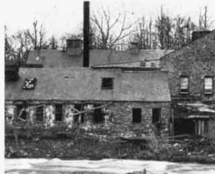
Cradle of the Iron Industry, on the site of the old Forge, where cannon balls were made for the Revolutionary Army. This site is now 60 feet under the waters of the Jersey City reservoir.
