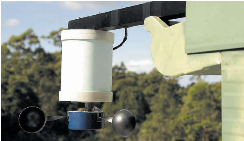
The working anemometer, seen positioned high on the roof. The cup covering the centre section of the rotating assembly was made from an aerosol cap. For improved durability, everything you see here should be painted.
