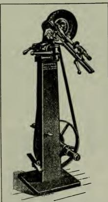
A Hand-controlled, Foot-operated Twist Drill Grinding Machine. The Drill is Revolubly Held in a Jig At the Correct Angle Against the Emery Wheel.
