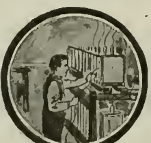
STORAGE BATTERY SYSTEM
