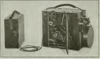
The Latest Gyroscopic Electric "Movie" Camera for Use in Photographing Battlefield and Aerial Views. The Gyroscope Holds the Camera Steady at All Times.
