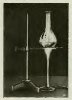
Fig. 91. Experiment No. 101, in Which Sodium Hydroxid Is Produced by Heating a Solution of Water, Slaked Lime and Sodium Carbonat.
