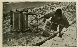
Welding Trolley Track Bonds With An Electric Furnace of Special Design. It Works Quickly and Is Portable. Time Per Weld Is About One Minute.
