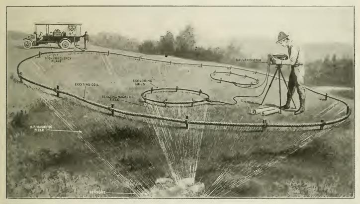
The Latest Feat in Mining Engineering is the Exact Location of Underground Metallic Ores by Means of Induction. The Largin Excited by a High Frequency Current from a Portable Dynamo Outfit. The Magnetic Field Created Affects the Ore Body, Reacts on the Smaller Exploring Coils and Indicating Instruments. arger Coll dy, Which
