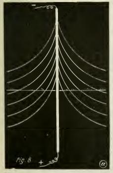
Diagram Showing How the "Wave Motion" About a Charged Wire Produces Concentric Rings of Force on a Plate Containing iron Filings. By the Upward Movement of the Conductor Currents.
