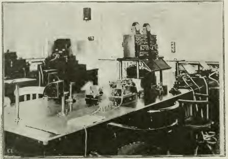
Photos from Donald McNicol Fig. 1. What the Interior of a Modern Ocean Cable Office Looks Like. This is the Trans-Atlantic Cable Office at Penzance, England, the No. 1 London Wire, Duplexed, and Creed Automatic Cable Instruments Being Shown.
