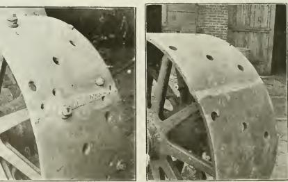
A Good Example of Welding Rolled Steel. The Rim of this Motor Truck Wheel is Formed by Rolling a Steel Plate Into Shape, Welding the Two Ends Together. The Illustration Shows it Before and After Finishing. The Metal at the Weld Was Cut Down Until It Was No Greater In Thickness Than That In the Plate and Still It Was Sufficiently Strong for this Severe Service. Finished Rim at Right.
