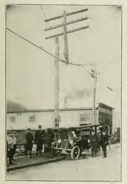
A Pecullar Accident in Which a Telephone Pole Was Severed By An Auto Crashing Into It. The Pole Remained Suspended by Its Own Wires.
