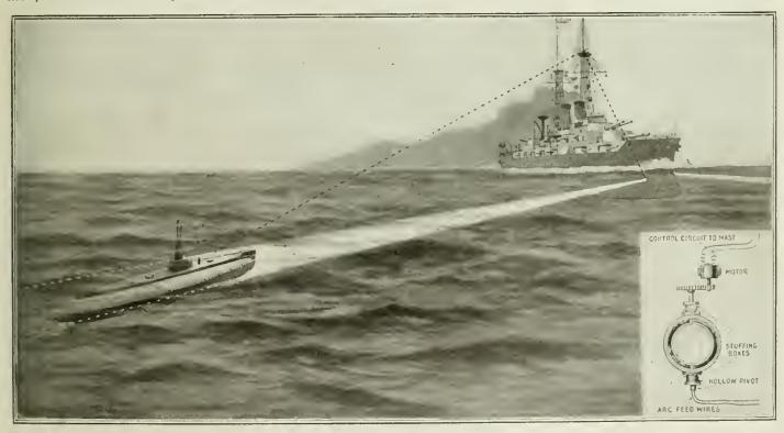
Why Not Locate the Submerged, Yet Always Dangerous, Enemy Submarines by Continually Flashing a Powerful Red Searchlight Beam Back and Forth Thru and Under the Water, Asks a Yankee Genlus. Once a "Bulge" is Spotted (Day or Night) in the Light Beam, the Observer on the Mast Signals That Fact to the Gun Crews. Consequence—as Soon as the Periscope Appears the Already Trained Guns Open Fire. The Spotting Range is Over Two Miles, Day or Night.
