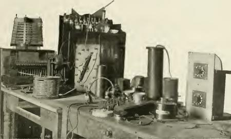
A Typical Radio Experimental Laboratory Equipt with a Variety of Condensers and Inductances, as Well as Other Supplementary Apparatus with Which Many Valuable Researches Can Be Made.
