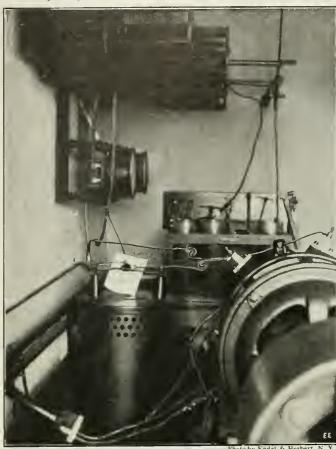
Our Uncle Samuel Seals Up Wireless Apparatus Tight When He Does the Job. A Heavy Wire Is Run Thru All the Binding Posts and Sealed as Shown, and Woe Be Unto Anyone Who Maliciously Breaks the Seal.
