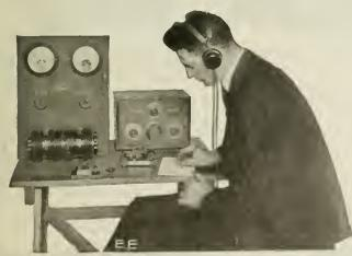
Fig. 3—Particularly Efficient Radio Set Well Adapted to "Mosquito Fleet" Service.
