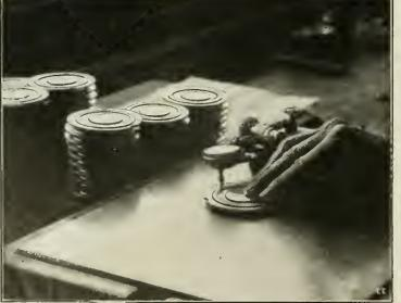
Manufacturing Quenched Spark Gaps in New York City for U. S. Naval Vessels. The Gap Plates Must Be Machined to 1/10,000 Inch Accuracy.
