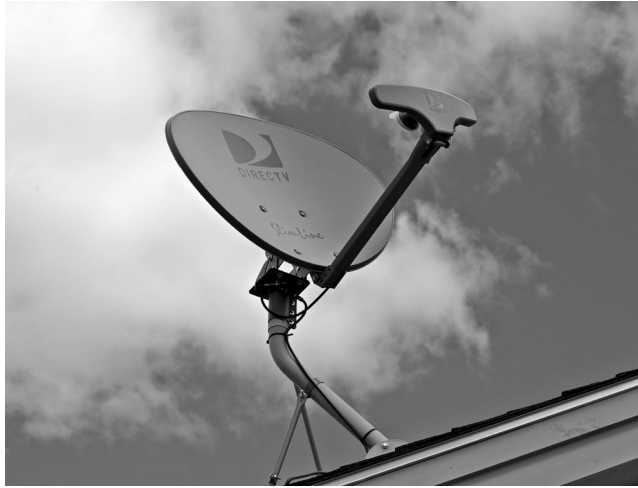
FIGURE 10-1 DIRECTV satellite dish with feedhorn.
