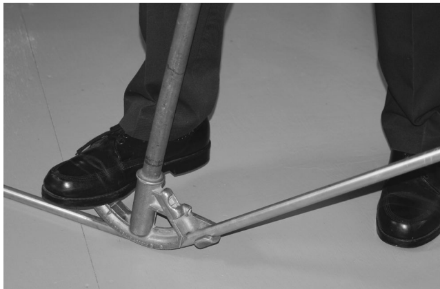
FIGURE 4-1 Bending electrical metallic tubing.
