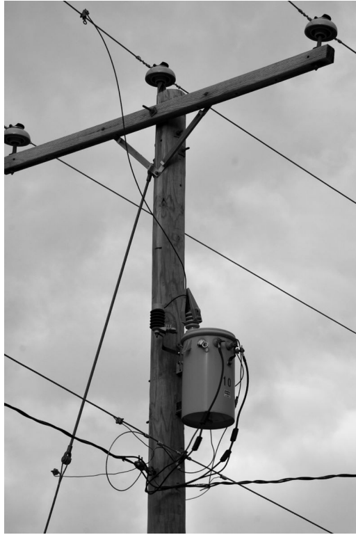
FIGURE 5-3 Single-phase transformer.
