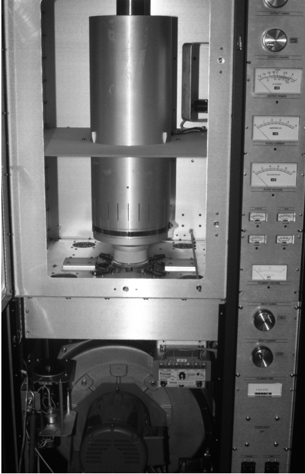
FIGURE 12.11 Clean the PA cavity assembly to prevent an accumulation of dust and dirt. Check hardware for tightness.
