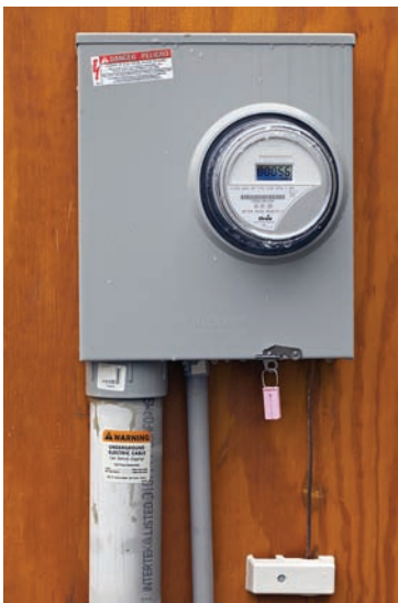
FIGURE G-11 The intersystem bonding termination, in the small white plastic enclosure below the meter socket, is a required part of every new service.
