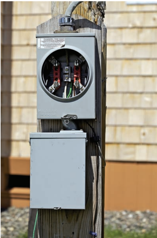
FIGURE 4-3 A temporary service. The two GFCI circuits need to be connected, and then it will be time to call the utility.
