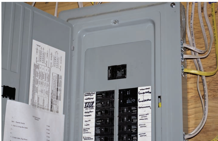
FIGURE G-12 The main disconnect is frequently located in the service-entrance panel.
