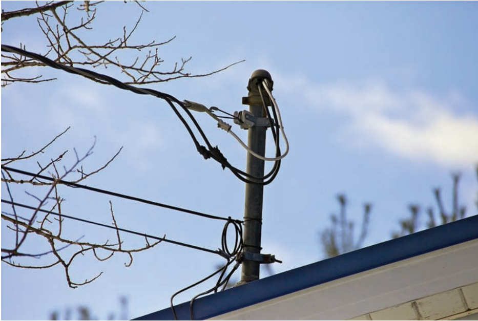
FIGURE 4-1 For this aerial masthead service, the point of connection consists of the crimped splices upstream from the weather head. (The cable TV and telephone cables attached to the service mast are a Code violation.)
