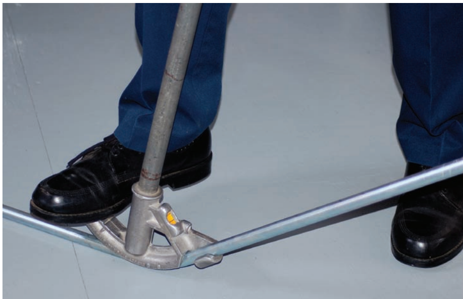
FIGURE 7-11 Bending EMT.
