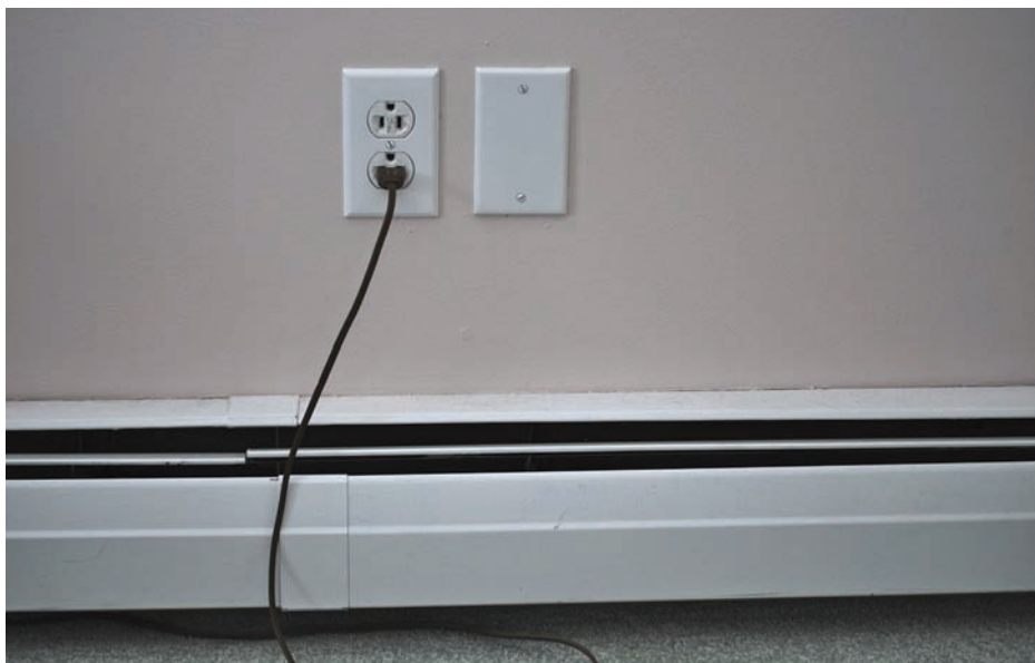
FIGURE 5-12 An electric baseboard space heater. The receptacle placed above it is a common listing violation because the cord is likely to enter the enclosure and be damaged by the heat.
