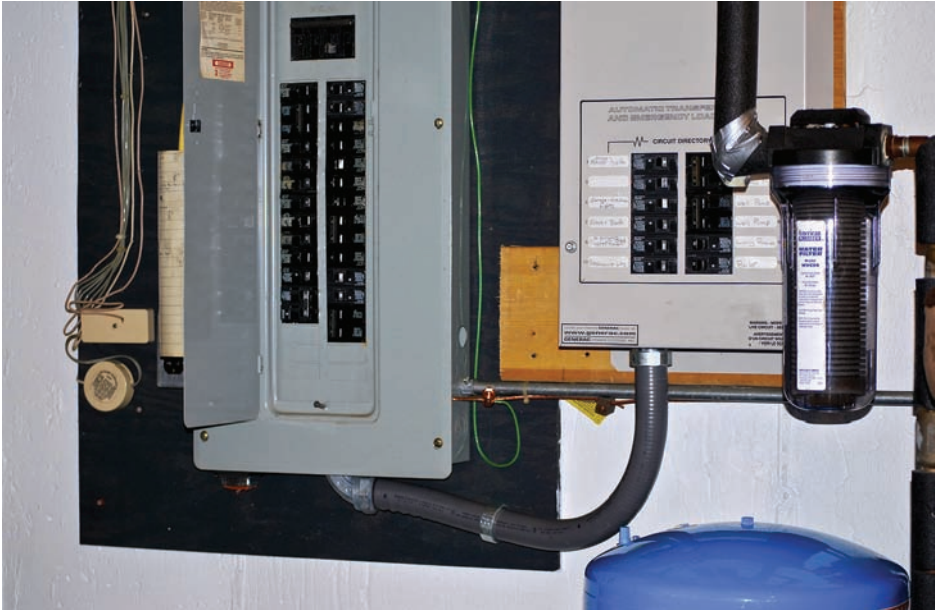
FIGURE 5-4 Note the clear violation of working-space requirements.
