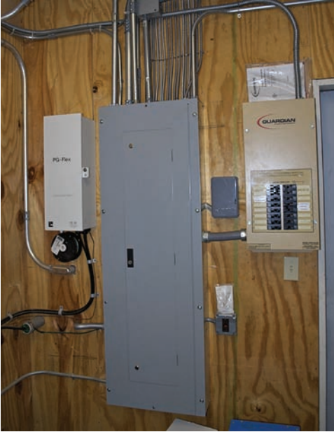
FIGURE G-20 A limited number of selected circuits are chosen to be energized by the alternate power source during a utility outage.
