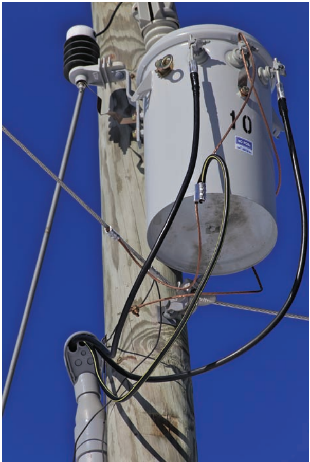
FIGURE G-21 A pole-mounted transformer connected to the service for an individual home.
